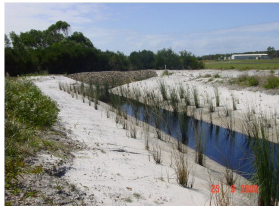
Figure 3 - Constructed retention Basin
